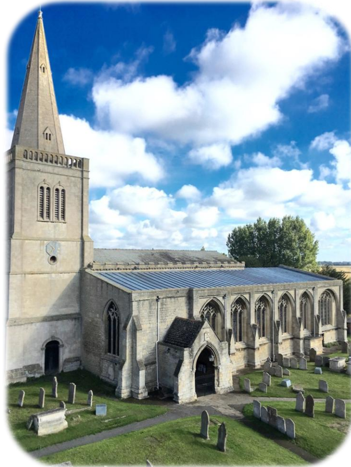
Photograph: © Chris Halley 2018
